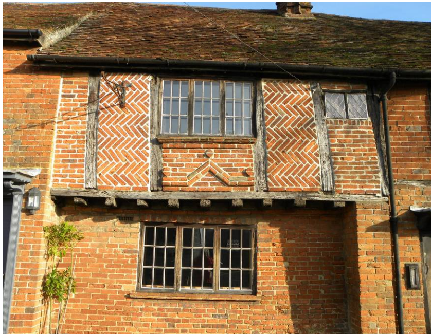
Figure 29: Brick nogging and jetty at 28 High Street
