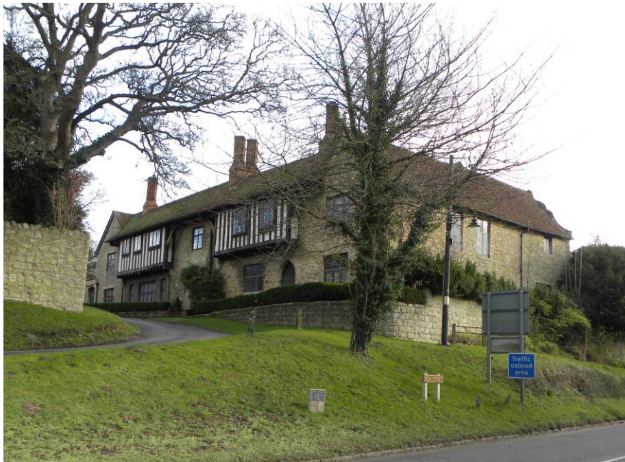
Figure 25: The Old House viewed from High Street
