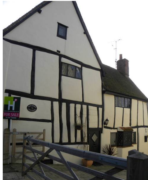
Figure 28: Close-studding at 53 High Street
