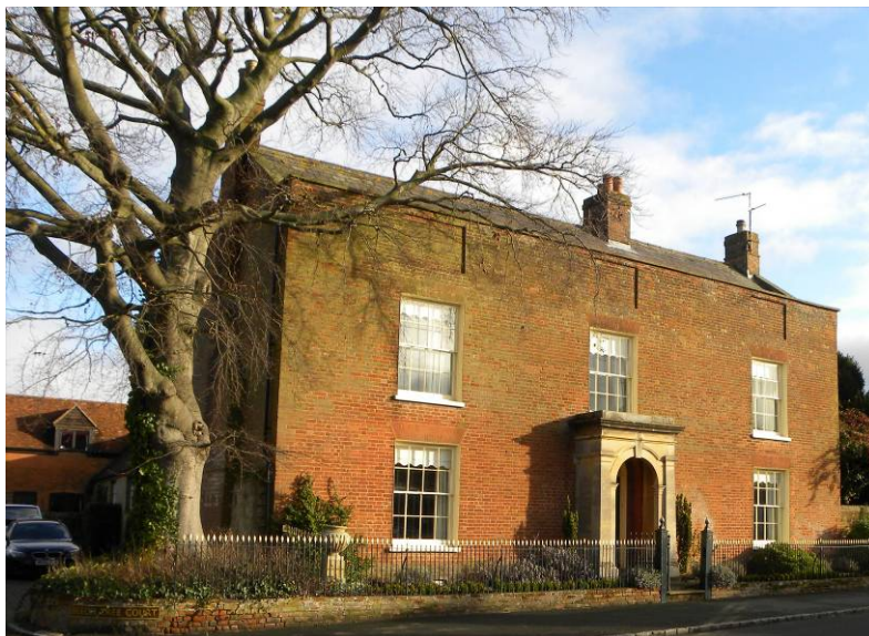
Figure 30: Beechmoor, 26 High Street
