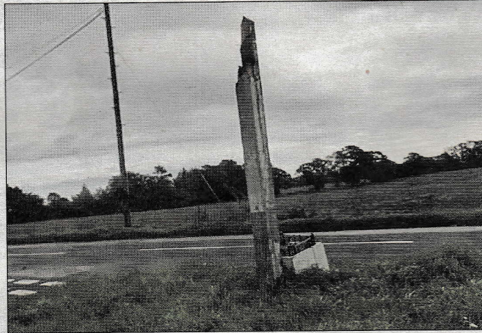
SIGN OF TIMES: The junction sign post at Inworth Lane has been left dilapidated
