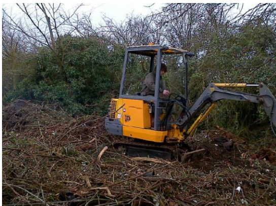
Clearing the site
