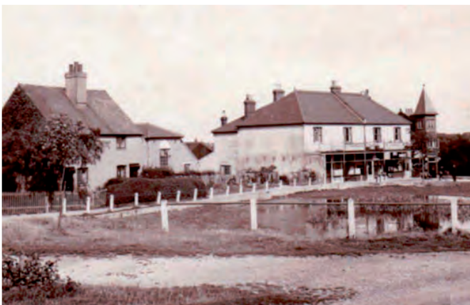
Westmore Green - historic photo showing shops and village club
