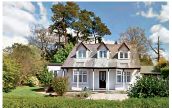
Examples of houses on Ricketts Hill Road
