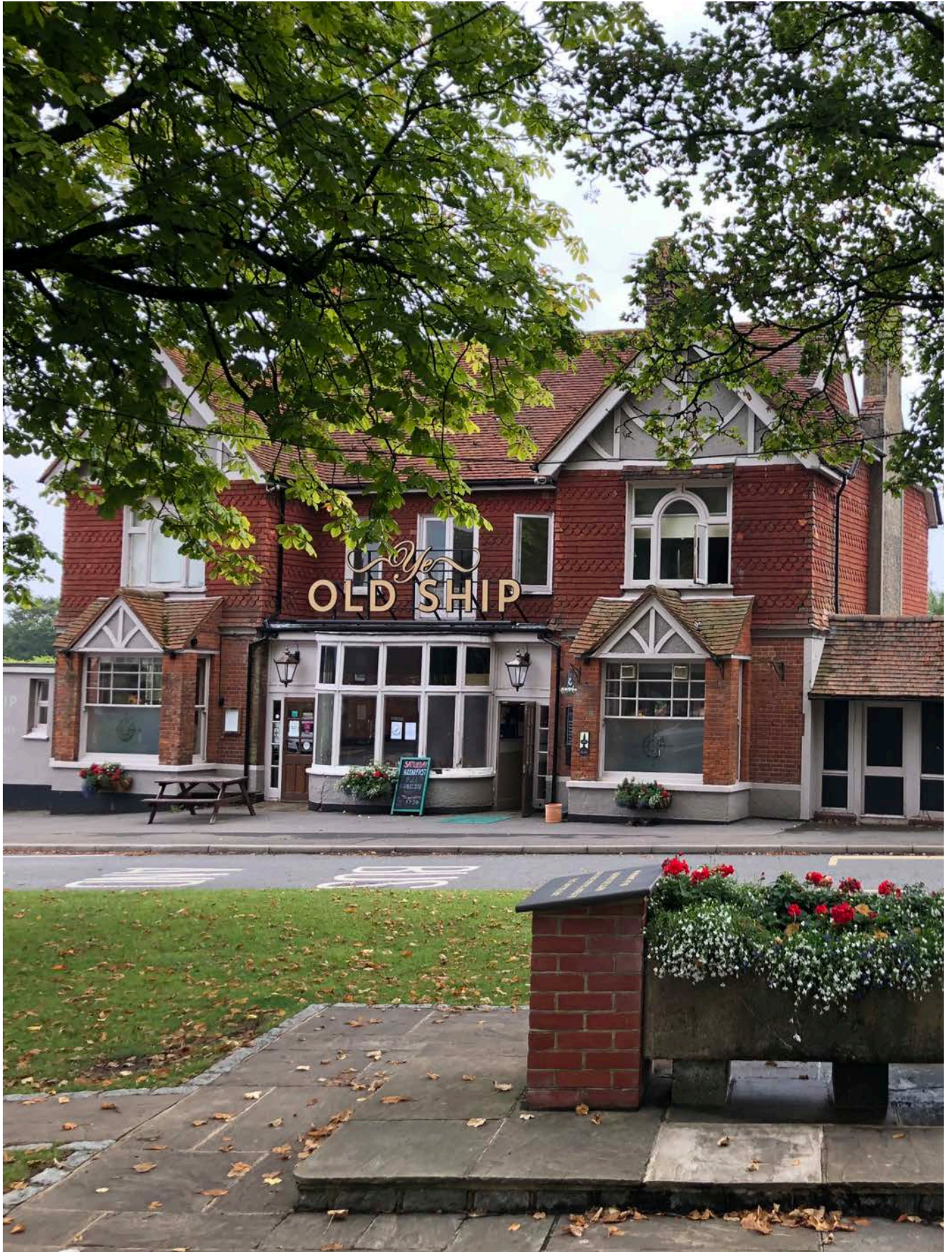
The Old Ship Public House with the war memorial stone in the foreground
