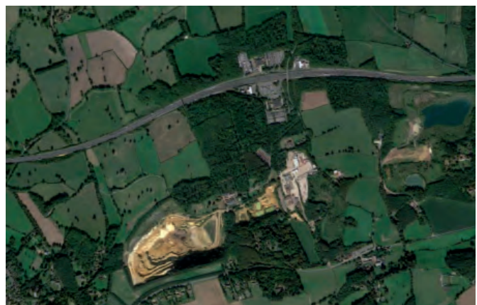
Clacket Lane Services and Moorhouse aerial view
