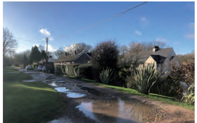
Maesmaur Road - localised flooding on unmade road after rainfall
