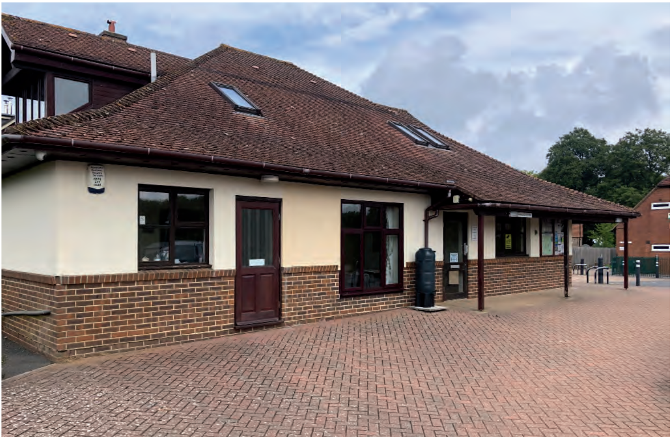
Offices spaces and the parish room at the Aileen McHugo Building
