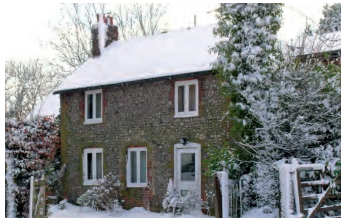
Traditional flint faced cottage with brick detailing
