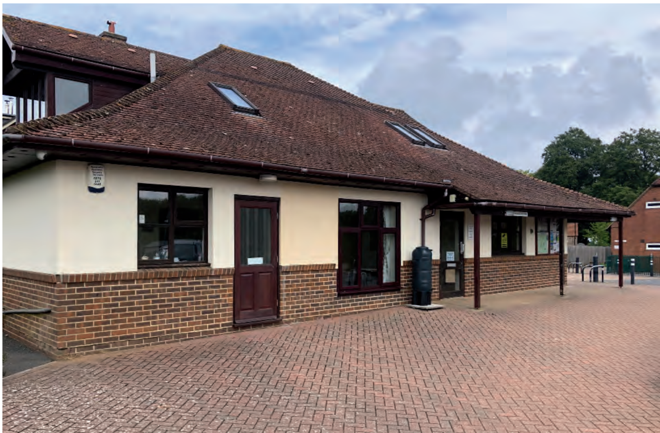
Offices spaces and the parish room at the Aileen McHugo Building
