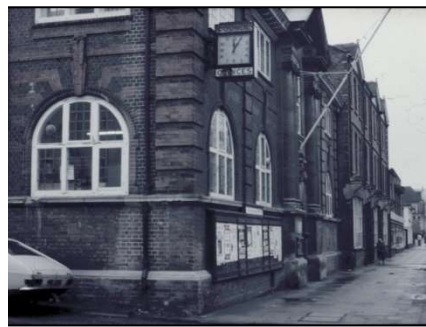
Frimley and Camberley UDC Offices, London Road
