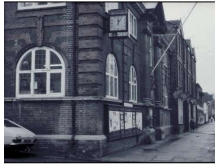
Frimley and Camberley UDC Offices, London Road
