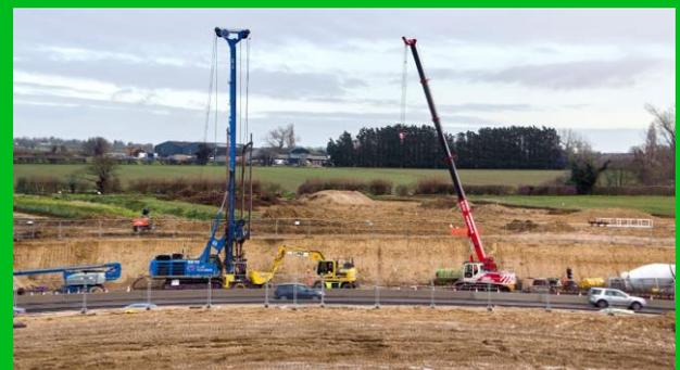
Piling Works Taking Place on the M11 Embankments
