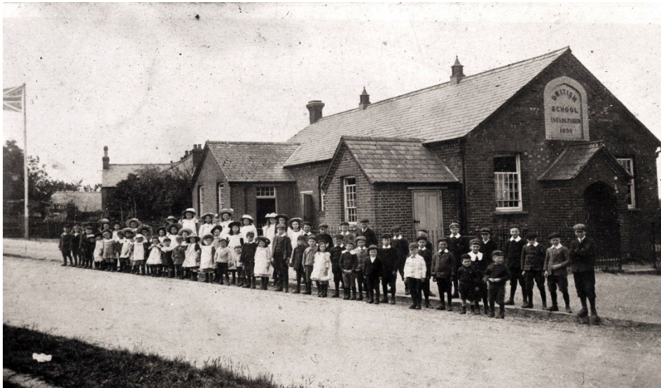
Another from post-WWI, showing improvement to the road verge
