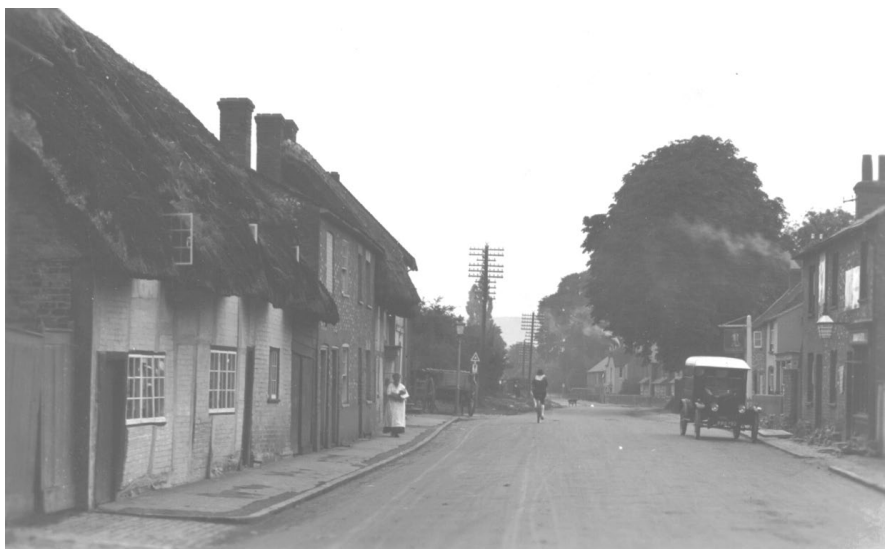
Bell Street, Princes Risborough, in the 1930s, looking West
