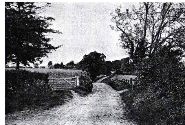
The lane to Wilderness Farm viewed from The Crossways, just before construction of Onslow Village commenced in 1920. The farmhouse is just visible amongst the trees.
