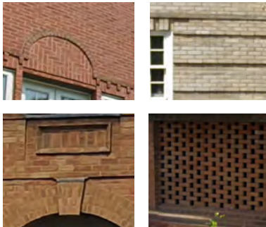
Brick Detailing (particularly around doors and windows but also contrasting panels)
