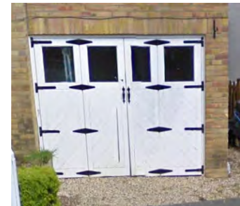
Garage doors should be painted timber or stained naturally. The level of detailing should reflect that of the dwelling
