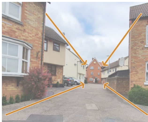
Vista terminated by a landmark building
