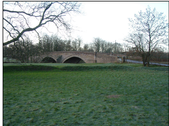
Plate 2. Musgrave Bridge showing the west end of the earthen dyke on the south side of Musgrave Church Field
