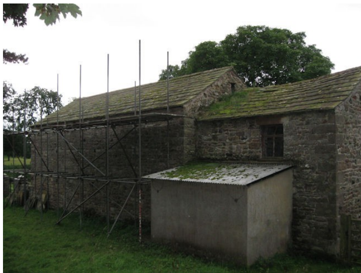
Rear (east) elevation showing former byre with 'modern' lean-to building.
