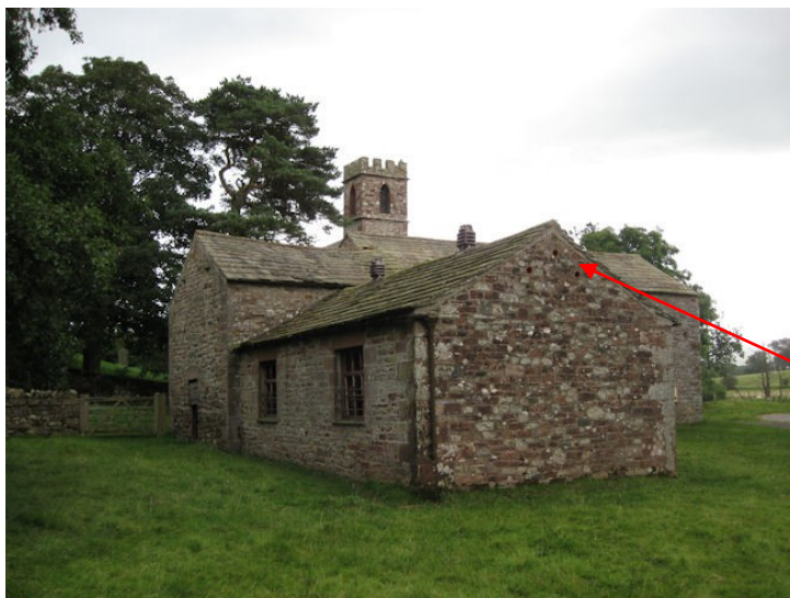
Rear of former stable annex adjoining barn showing West gable wall with round ventilation holes (red arrow) in the upper section of the wall
