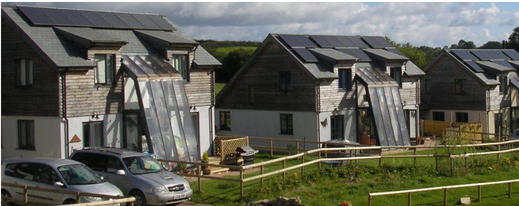
Broadhempston CLT, Devon
