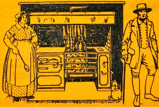
Early Nineteenth-century Carbon Range
