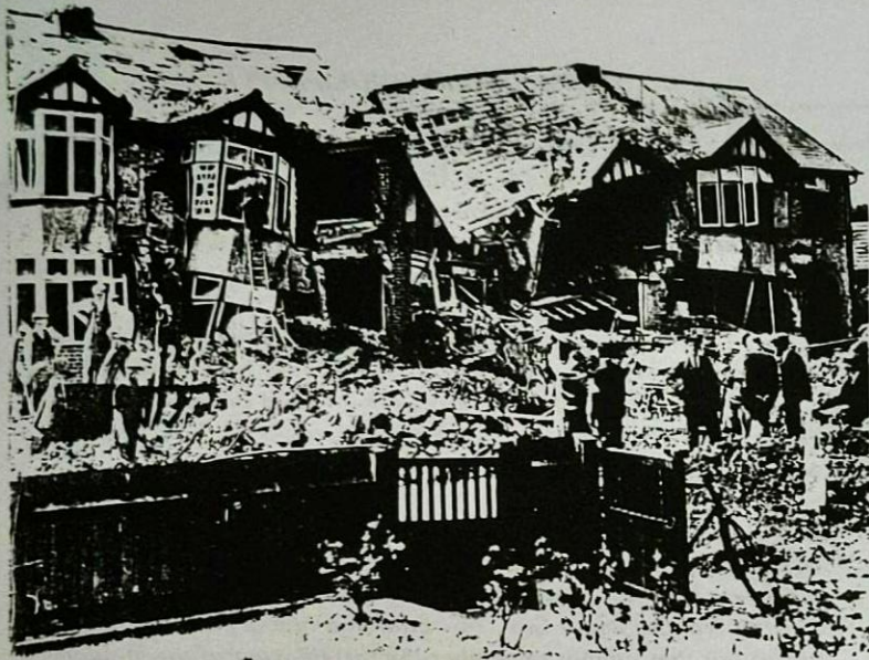
Houses damaged by a flying-bomb, Fambridge Road, Maldon (September 20, 1944)
