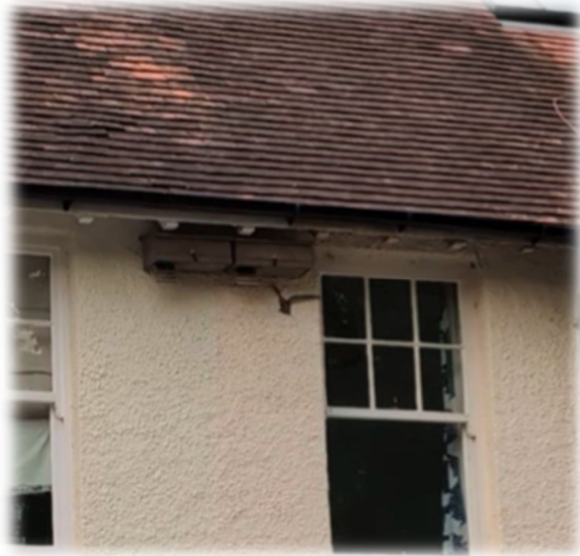
The moment just before entry at one of the boxes in De Montfort Road.
