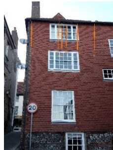
St. Swithun's Terrace
