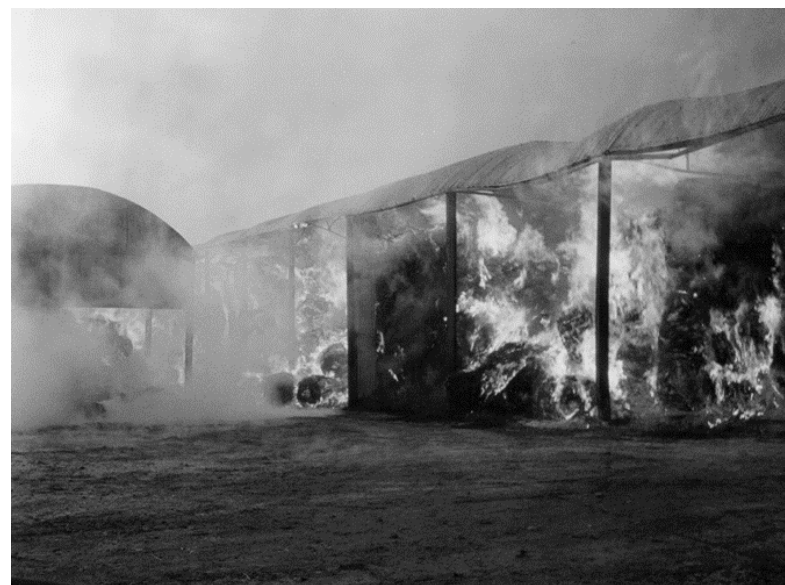
Figure 2. Barns on fire at Leaden Hall Farm—date unknown
