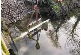
In December 2019 upstream works began on site and continue. Riverbed material is being moved upstream where it will be spread to the desired level. The photo at the top of the column shows the floating platform and equipment used to lay the materials in the riverbed.
