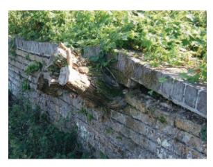
The platform had fallen into a pitiable state of neglect, with roots growing through the engineering bricks, and the platform crumbling under the invasion of ivy and other creepers.
