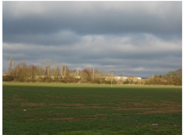
CML buildings from Ulting Lane
