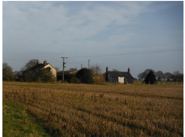
Dilapidated buildings (Braintree District)
