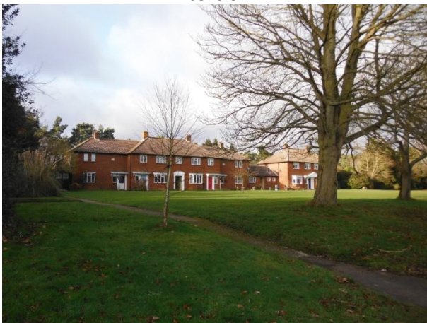
Waterworks houses in Ulting Lane
