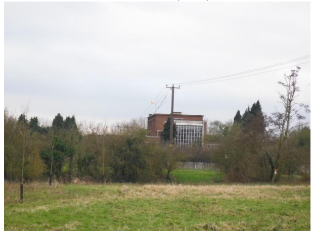
Langford Treatment Works
