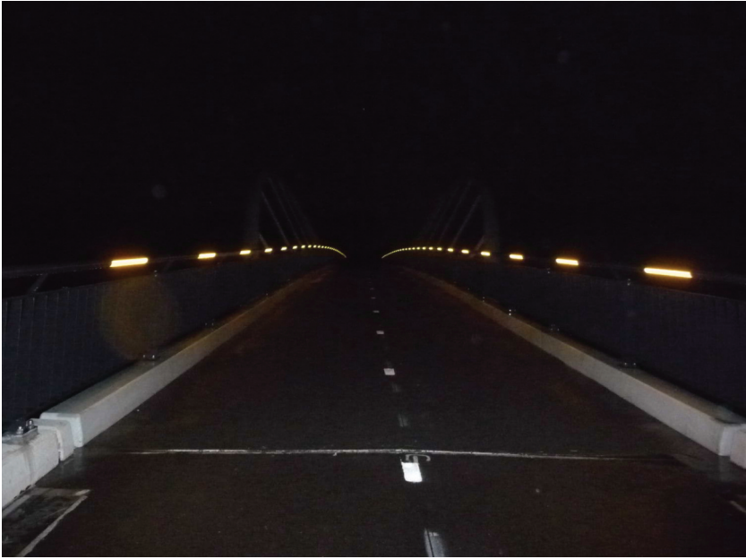
FIGURE 7. Narrowband amber handrail lights over the A74 bridge at Tegelen, Netherlands.
