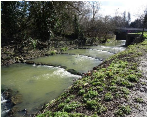
Photograph 3 River restoration: knocking out weirs, Hogsmill River A3, 2015
