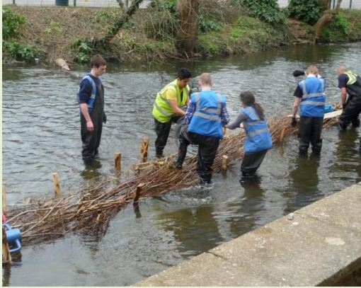
Photograph 1. River restoration: narrowing the channel, Hogsmill River Knights Park, 2014
