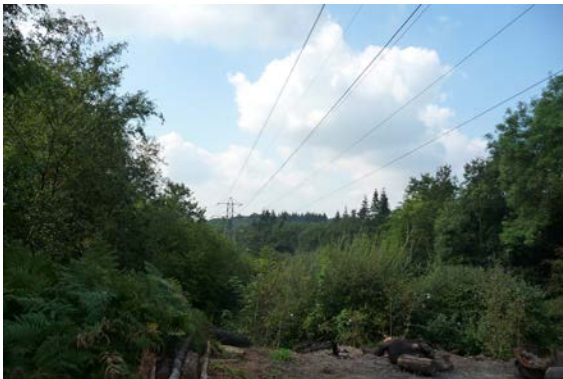
Photos: National Grid pylons, World's End
