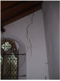
Since 2005 cracks have developed where these rooms join the main church structure. Lately further cracking in the North and South walls suggests that there are ongoing foundation issues related to the sub-soils.
