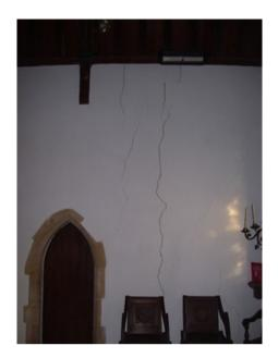
Our Architect has prepared a specification for the underpinning of the Vestry and North Chapel, together with high level tie rods to stabilise the East Wall, and the cost of these works will be in the region of **£50,000**.
