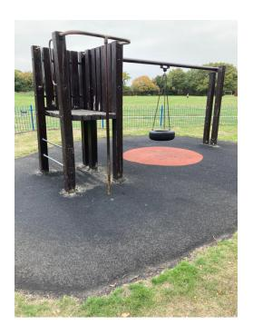
To replace old Fireman's Pole & Tyre Swing due to deterioration of wooden supports and because they no longer meet latest safety standards.
