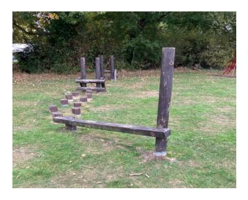
To replace old wooden Burma Chain Bridge and Balance Beams and Stepping Logs due to deterioration of wooden parts and safety issues with chains and replace with new more exciting "Trim Trail"
