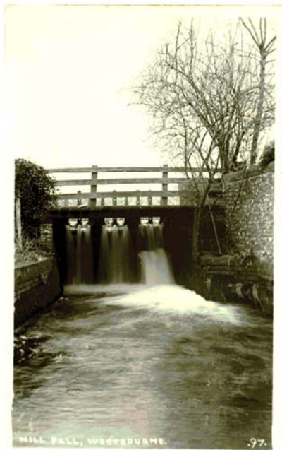
Westbourne Mill sluice – shows big vertical drop and 'challenge' to sea trout
