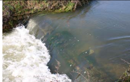
Weir recommended for modification or removal to restore chalk stream habitat – not central slots could be removed
