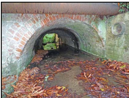
The brook culvert at the base of Sandon Hill
