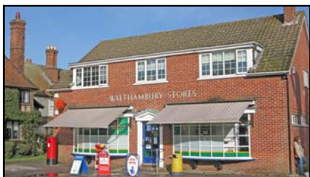
Walthambury Stores and Post Office
