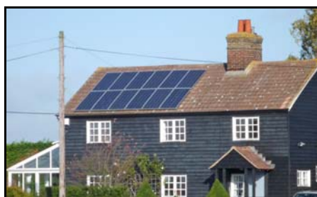
A solar panel installation
