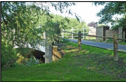
The bridge at Howe Street
