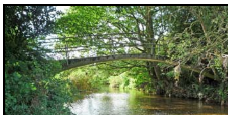
Cut Throat Lane Bridge
