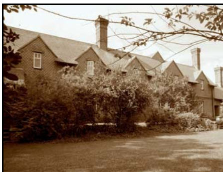
Church Housen Almshouses
