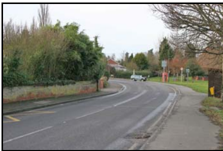
Roadside pavements on both sides of the B1008 in Ford End
