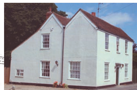
The Hoppit 18th c. timber framed & plastered
