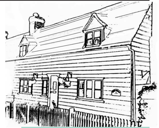
Small weather-boarded cottage South Street
