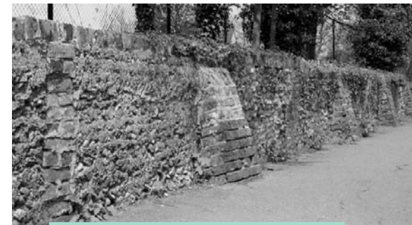
Flint wall with brick buttresses, South Street
