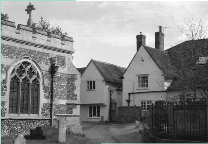
The churchyard and rear of Six Bells Cottages
