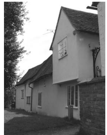
Rear of cottages that formerly faced the churchyard
