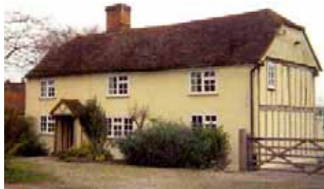
Green Oaks after extension
