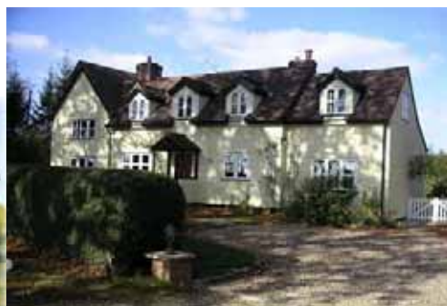
Cottage with gravel driveway and hedge boundary
