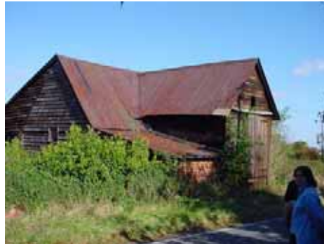
Old timber barn in Black Chapel Lane
