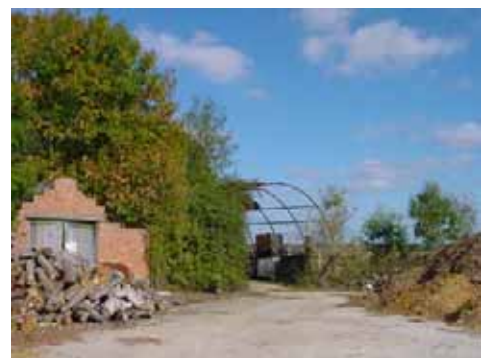
Derelict buildings near North End Place
