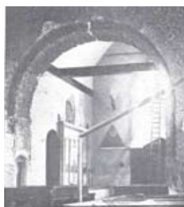
Roman bricks in the chancel arch at St Giles' exposed during the Victorian restoration
