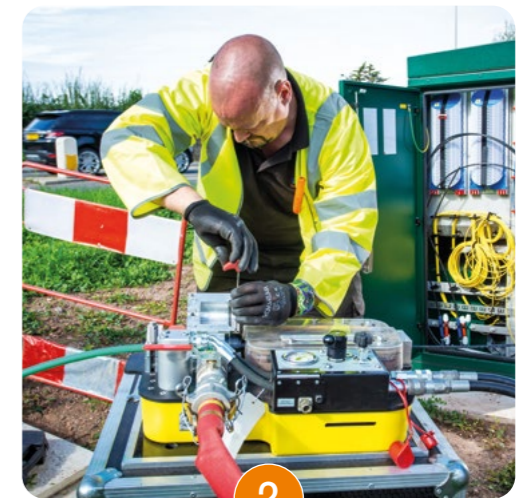
Fibre-optic cable is blown into ducting
