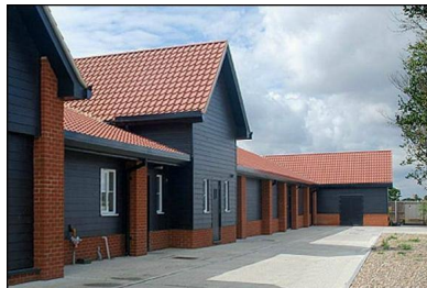
salt processing facility
