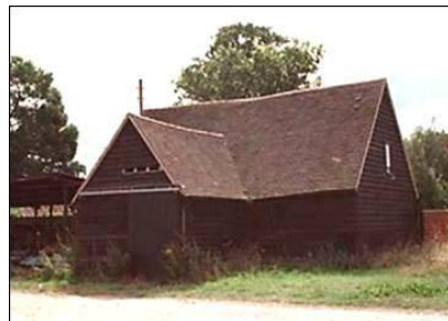
barn destroyed by a fire in the 1980s
