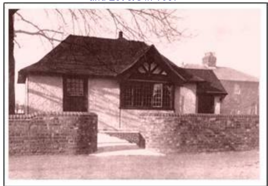
The Parish Rooms
