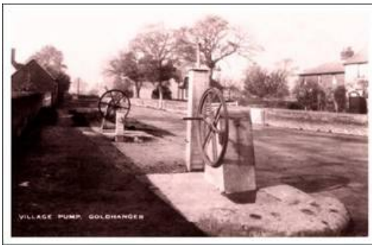
Two Pumps after a new well was dug
