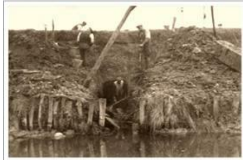
Removing the old sluice
