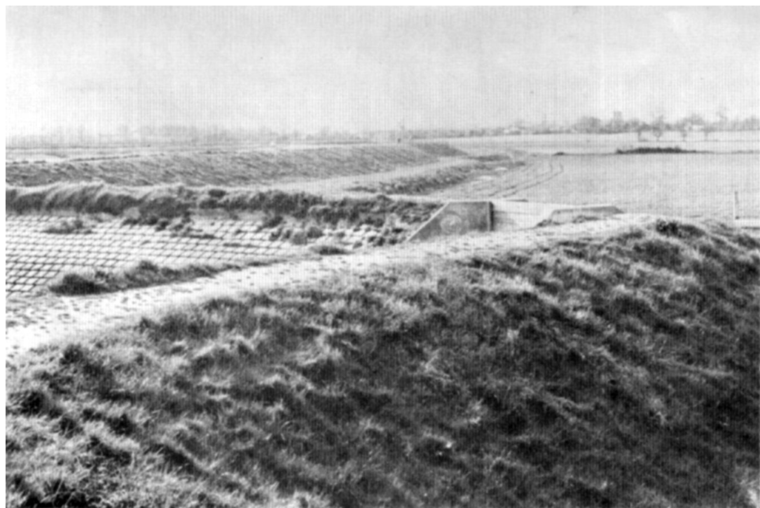
The sea-wall east of the creek today looking across the hatches and borrow-pit to the village with arable fields on the right
