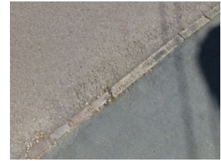
Stone and concrete kerbs line the carriageway
