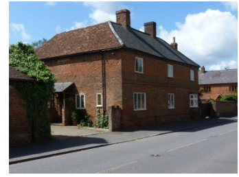
This unusual building has slate on the front roof slope, and tile on the side roof slope
