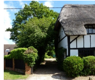
Views along the street and glimpses between buildings are important
