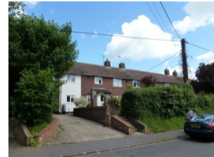
The modern houses on Spring Lane (9-23 odd)
