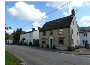
This steeply pitched, machine made clay tile roof indicates that the building may have been thatched
