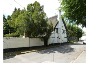
Tall ridges and low eaves are typical of thatched buildings
