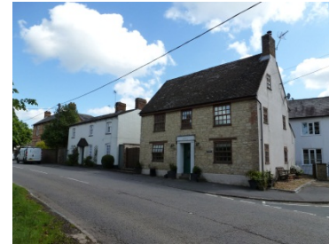
Historic buildings at the junction of Spring Lane and Winslow Road
