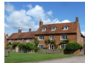
Traditional casement windows and small dormers are common
