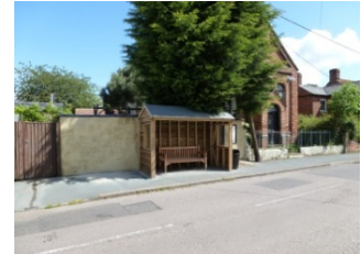
The bus shelter is visually unobtrusive
