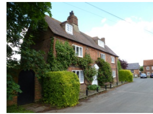
A typical, detached, single span house on School End
