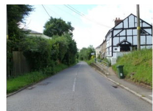
The road surface is lined with stone kerbs
