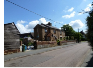
Ancillary structures are weatherboarded
