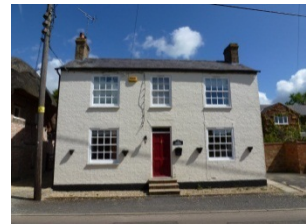
Traditional timber windows and doors
