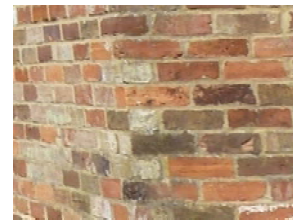
Brickwork in stretcher bond
