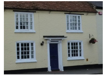
Decorative windows and doors surrounds are seen in this part of the village
