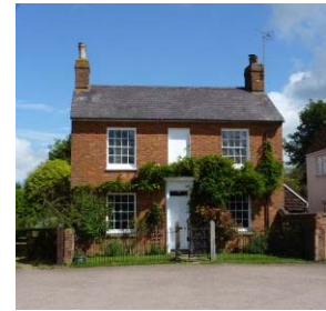
A typical 2 storey building on The Green
