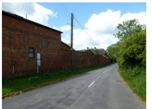
Buildings and walls line the street for most of its length
