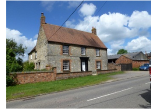
Stone with brick detailing and hand made clay tile
