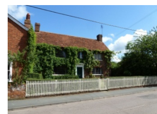
Traditional railings are found in this part of the Conservation Area
