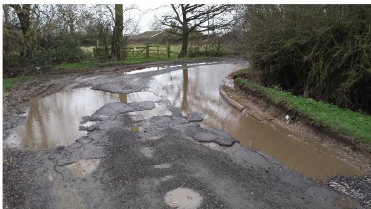
Plans to repair the failed road surface at the top of Spring Lane have been made. Last time we heard TfB were have engaged contractors and the timetable is now in their hands. The plan was for the work to start at the end of March or sometime in April. The road will have to be closed as work is quite extensive. Although heavy lorries are the primary cause of the problem, it is exacerbated by
