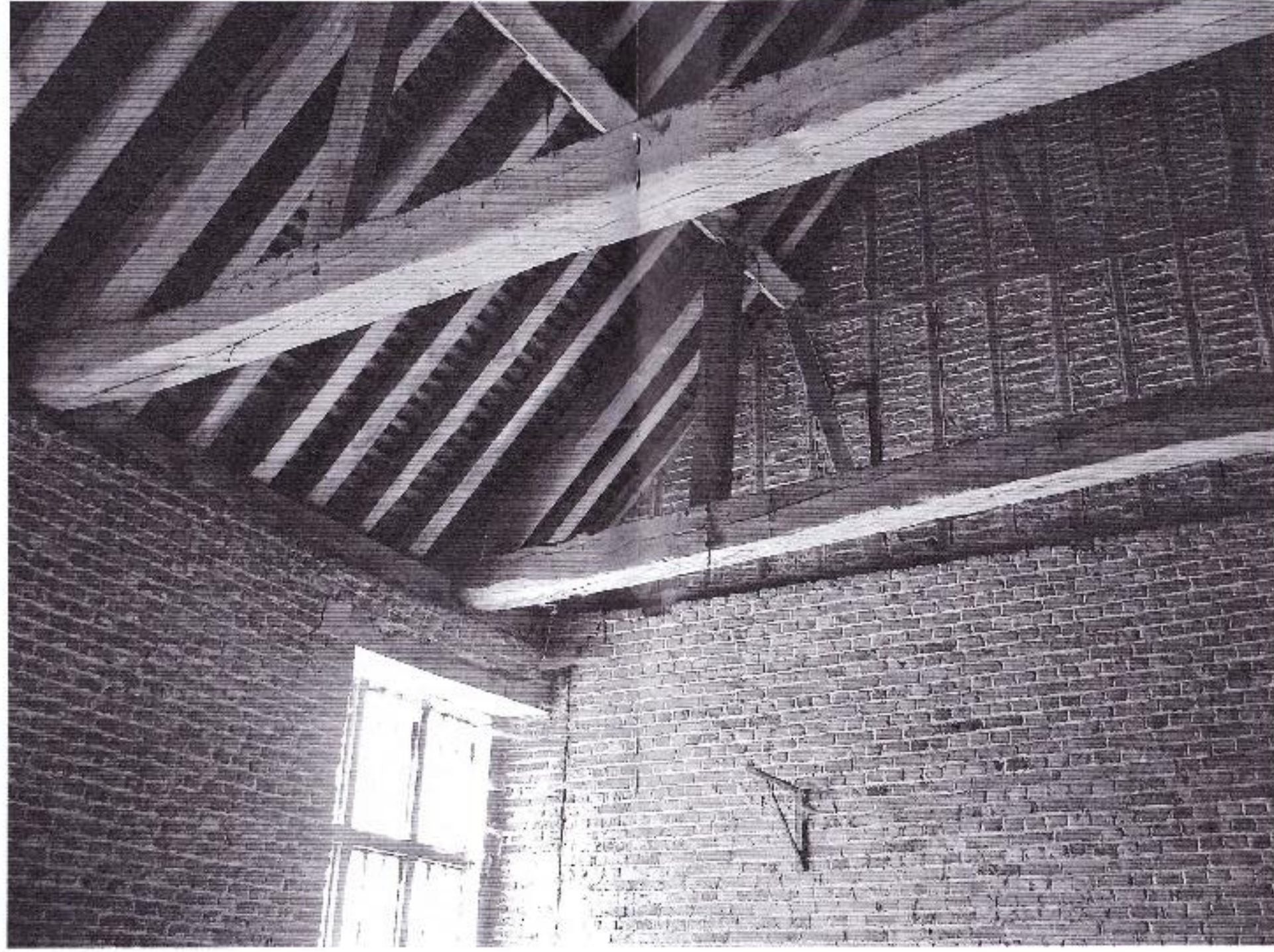
Beams in brick building of shop, Osterley Park, London
