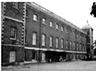
The north side of the House with four drainpipes visible.
