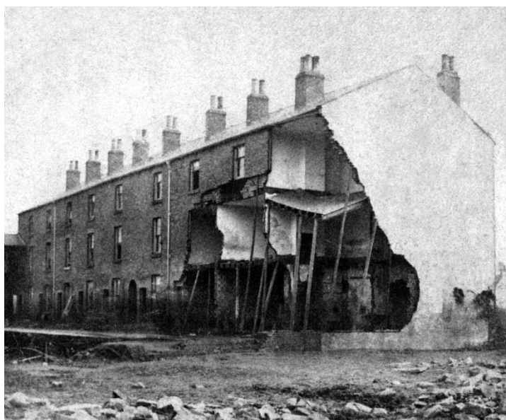
Brick Row, Holme Lane
