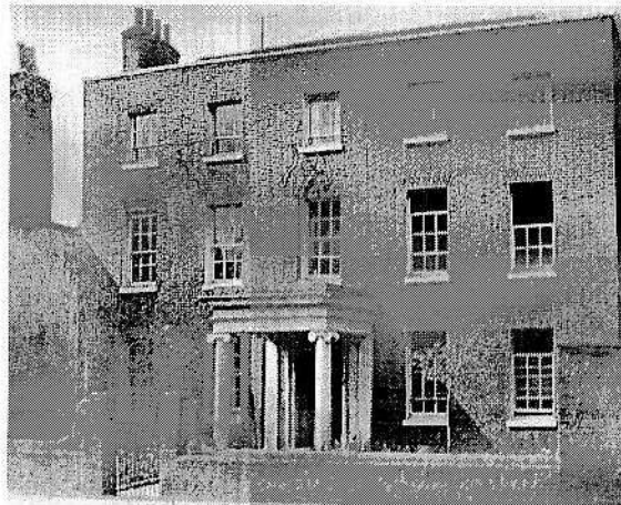
Allen House prior to demolition.
