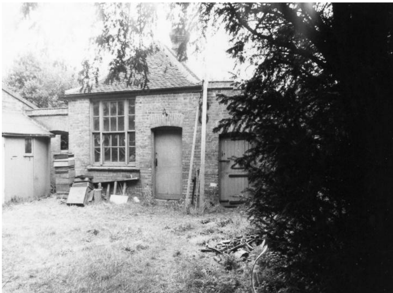
1980: The 17 th century brewhouse, converted to a laundry and bakehouse for the Victorian conversion, and latterly for our workshop, in 1980. To the right, with the stable door, is the coke/coal shed, originally the stable for the donkey who worked the well pumping gear. The site of the well shaft is out of shot, to the left.
