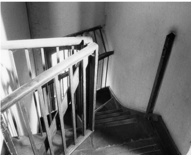
1980: Top of back stairs, the only access to the top floor, and lit only by the long window below the turn in the stairs. The nursery gate guarding the staircase is original, and still present in the converted building today
