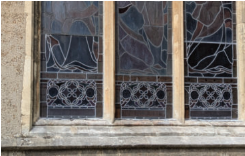
Same window after restoration
