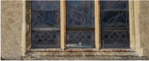
Lower part of a window prior to restoration
