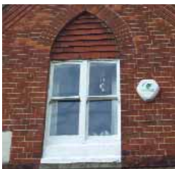
Original windows in the Victorian former rectory.
